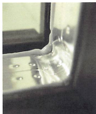
Figure 3: Primary Sealant (gray) at Bent Corner
