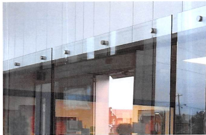
Figure 4: Example of point-supported glass barriers with thru-hole fittings.
