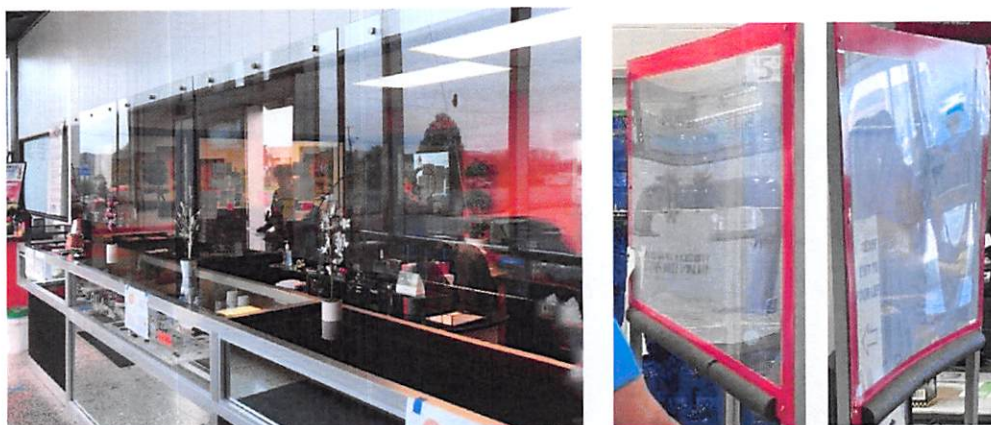
Figure 1: Safety glass installed for personal protective barriers (left photo) can provide a sleek, professional, sanitary, yet welcoming feel for consumers entering retail stores compared to plastic barriers (right photo) where rough edges and hazy distortion combined with surface scratches detract from the consumer experience and collect dirt and potentially bacteria.
